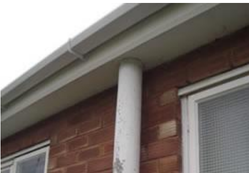
Asbestos cement drainage pipe (downpipe)
