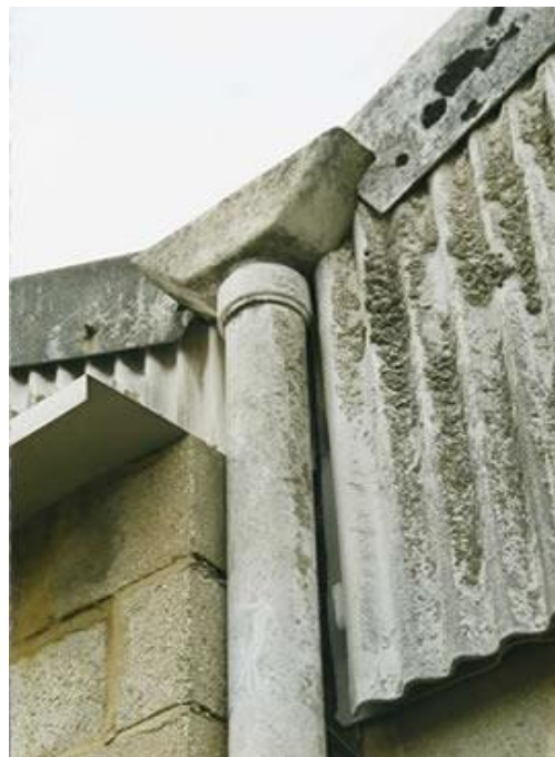
Asbestos cement downpipe, hopper and profile sheet
