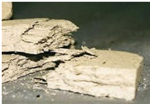
Pieces of Asbestos Insulating Board (AIB)
