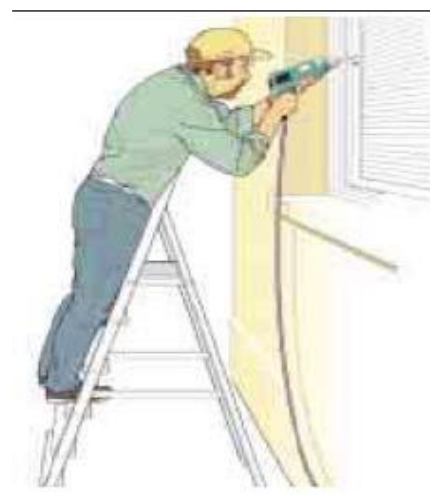
Correct – steps facing work activity
